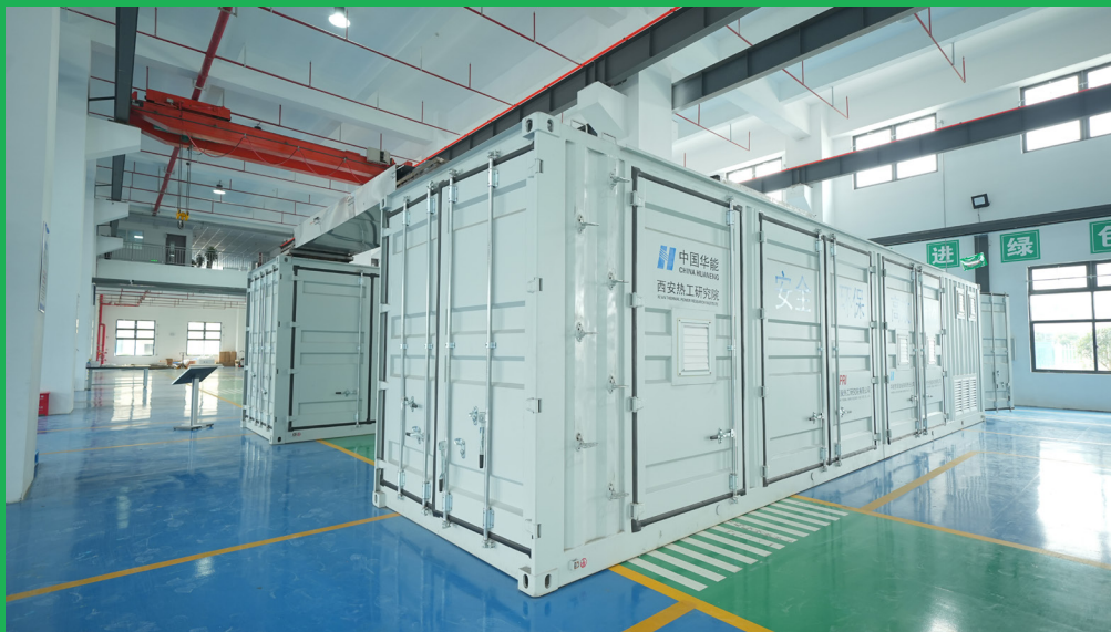
China Huaneng Group Co., Ltd. Fujian Luoyuan Power Plant, 200 kW / 400 kWh Metal-free flow battery system, frequency regulation project
