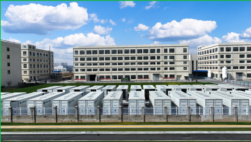
5 MW / 20 MWh metal-free flow battery system for long duration energy storage
